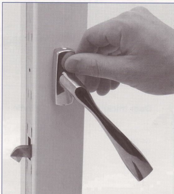
The cover plate is pressed into place. Mounting is finished.
